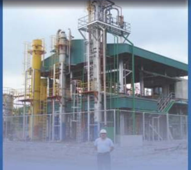
A FENIX-SHUTEK BIODIESEL PLANT COMMISSIONED BY US
